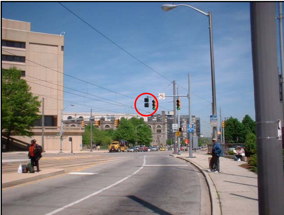
Light Rail Signal: Howard Street northbound at MLK Boulevard crossing railroad tracks
